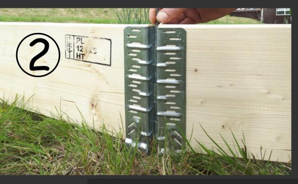
Align the hinges and secure them with the wire. Use a hammer and drive in the wire all the way in.
